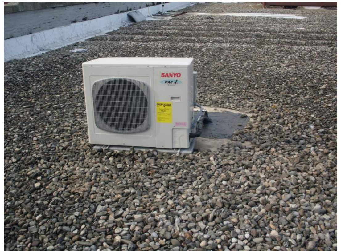
ROOF TOP INSTALLATION OF OUTSIDE DUCTLESS UNIT CONDENSER
