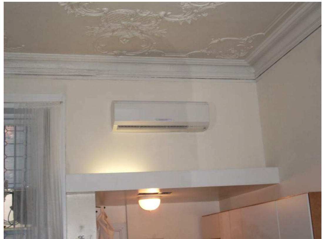
WALL MOUNTED DUCTLESS UNIT
