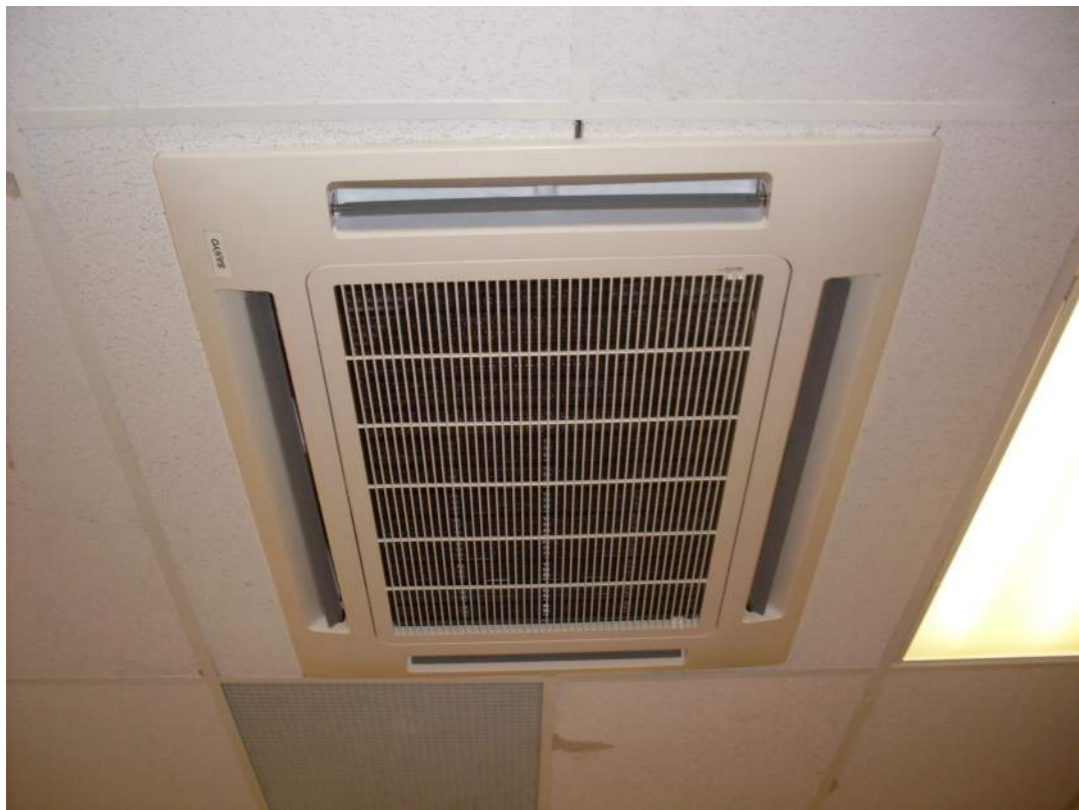
CEILING MOUNTED DUCTLESS UNIT
